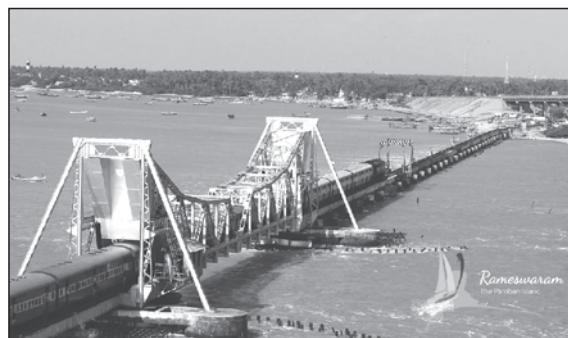
The Pamban Railway Bridge connecting the island
